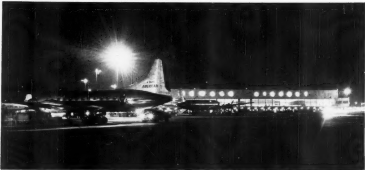
RAMP at Newark Airport at night has in background three-year-old passenger terminal, already short of ticket counter space. The airport, regaining its place in the New York metropolitan area, handled almost 2 million passengers in 1955.
